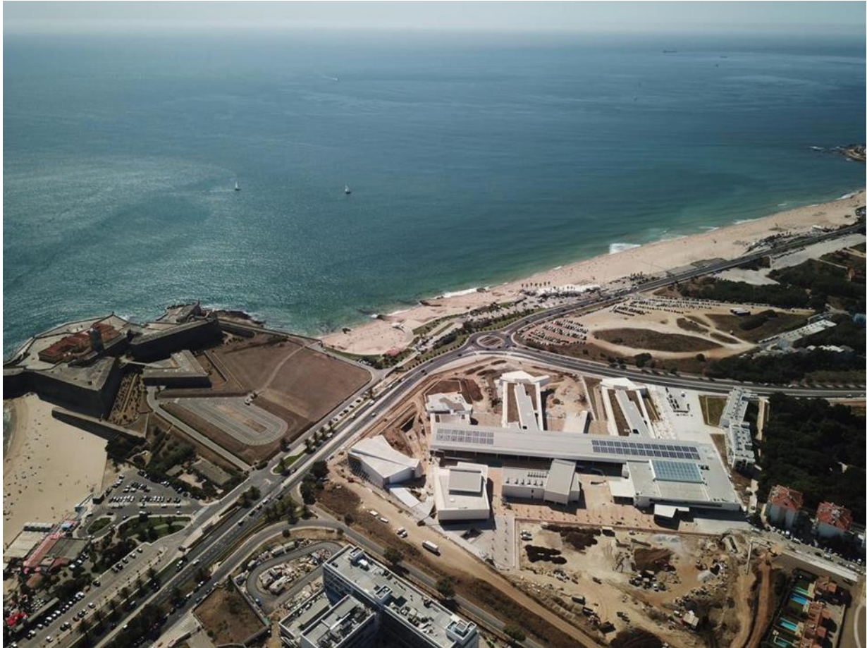
Figure 1 - Aerial View of the NOVA SBE Campus
